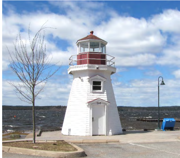
Lighthouse at the Renforth Wharf, Rothesay- New Brunswick
